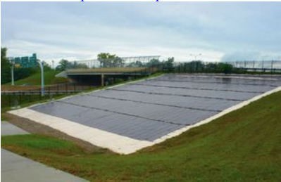
thin-film PV panel / amorphous silicon LANDFILL
