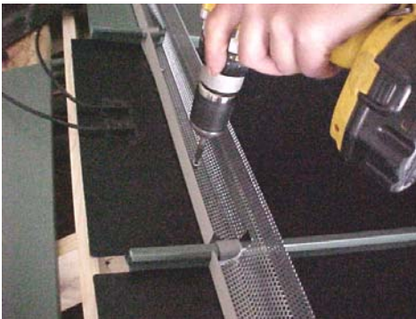
Installing Z-Closure, taking care to put screws through areas where penetrations are allowed
