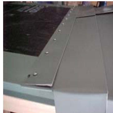
Installation of Starter Cleat
