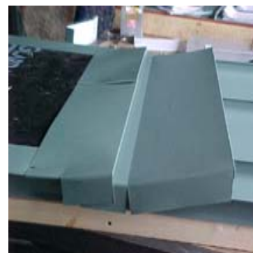
Head flashing after assembly
