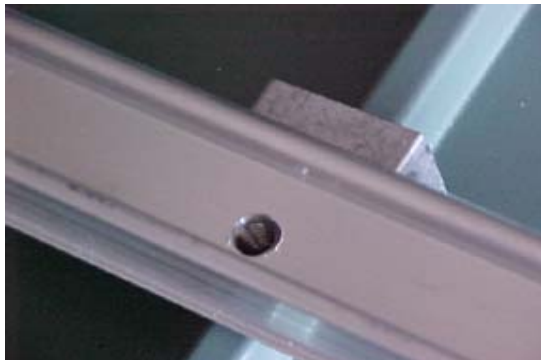
Hole Drilled in Channel
