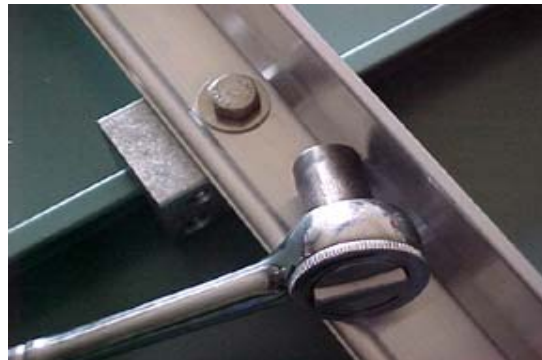
Channel Fastened
