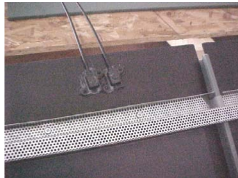
Installed Z-Closure, ready for quick connection
