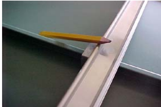
Snow Guard Channel in Place
